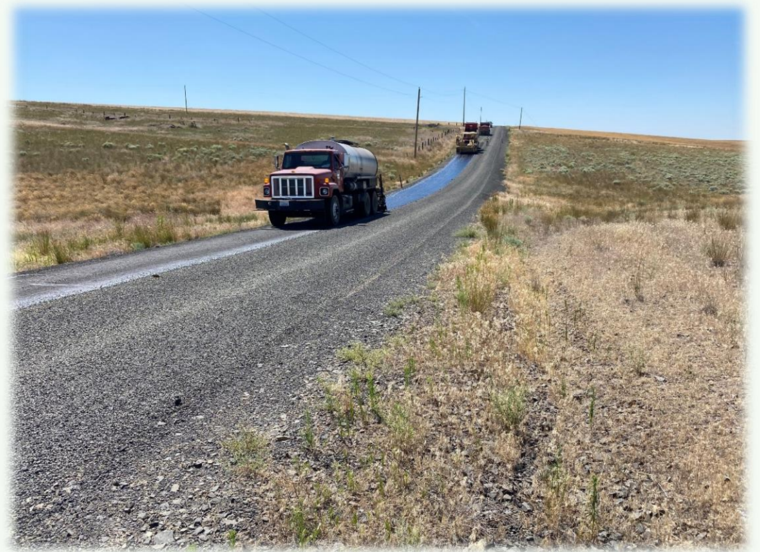
Bituminous Surface Treatment in Progress
